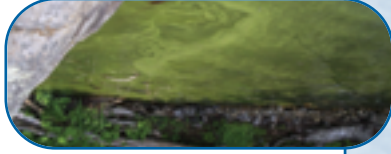
Paint spill aspect
